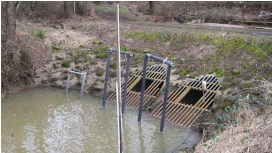
Figure 34. Upstream view (upper panel) and downstream view (lower panel) of antenna configuration at the SWCS array, which was operational during 2014–2016.
